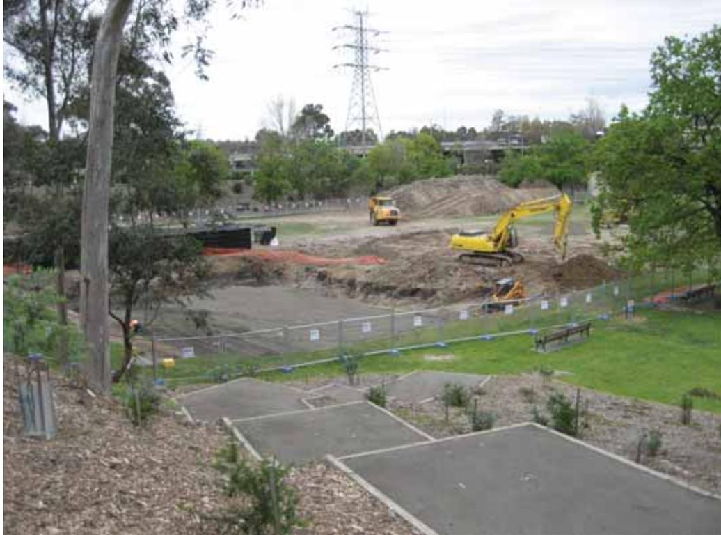
The stormwater and reclaimed water storage tank being built under the McKendrick Oval
