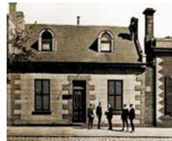
FIRST SITE – 1851 155 Spring Street, Melbourne
