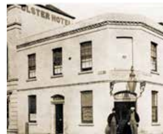
SECOND SITE – 1851 61 Spring Street, (corner of Spring and Little Collins Streets, Melbourne)
