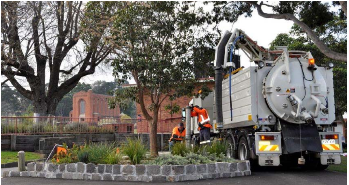
Cleaning drains near the Chapel.
